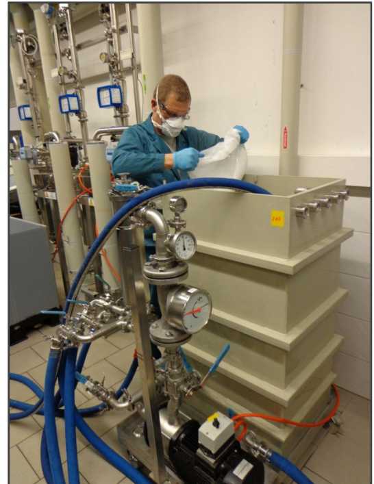
Employees applying chemicals for passivation.
